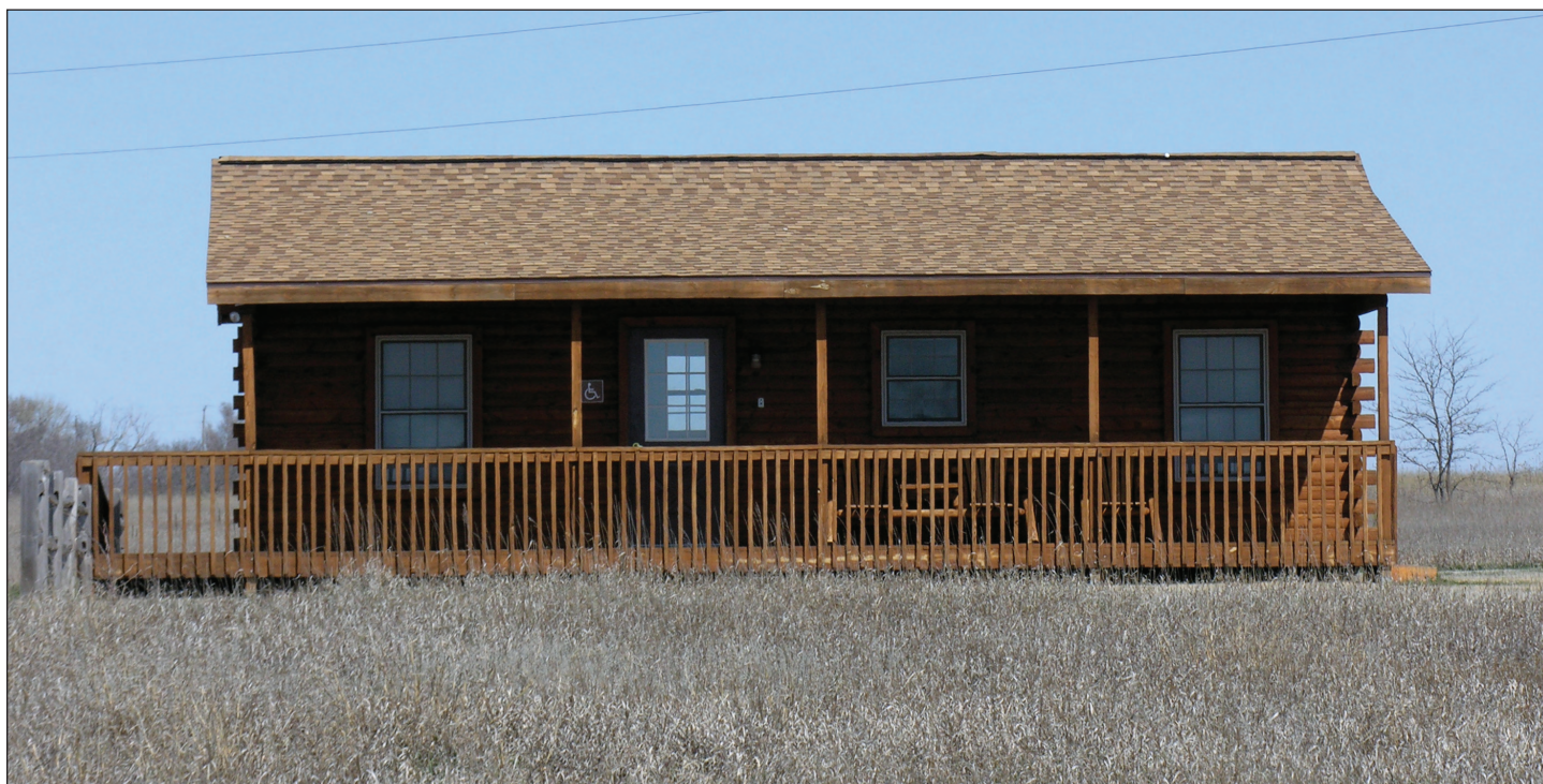
This rental cabin was added last year and has been popular with park patrons. Another cabin is scheduled to be added this summer. Both cabins are deluxe, offering heating and air conditioning, full kitchen and bathroom and all the comforts for home.
